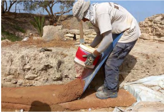
Laying hyper-adobe around soil scarp under Building W
