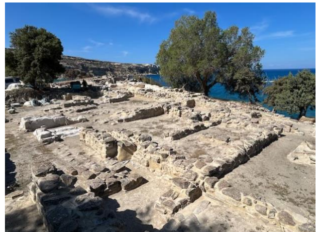
Completed stabilization of Hilltop Houses 2025
