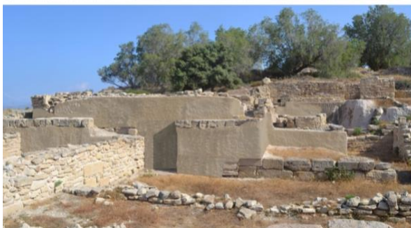
Figure 6. Scarps that will be restored after completion of pilot project to replace with new stainless steel or hyper-adobe embedded in facing mortar supported by new foundations
