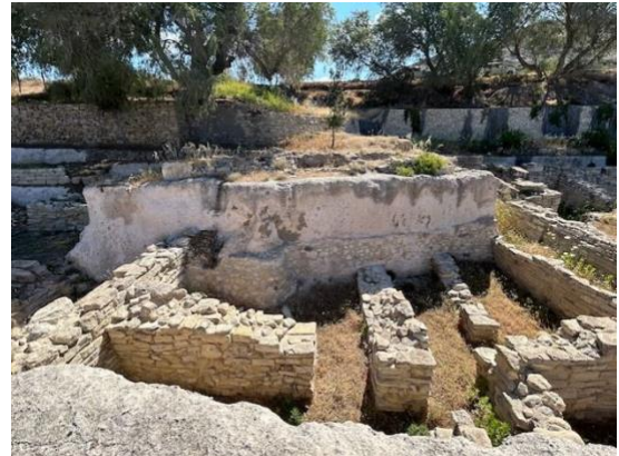
Terrace scarp north of Altar terrace showing foundations and eroding mortar facing
