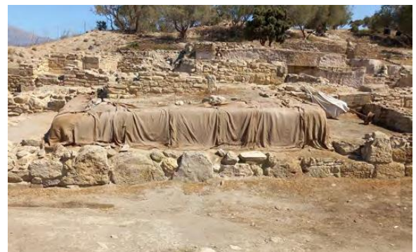
Curing hyper-adobe and mortar facing
