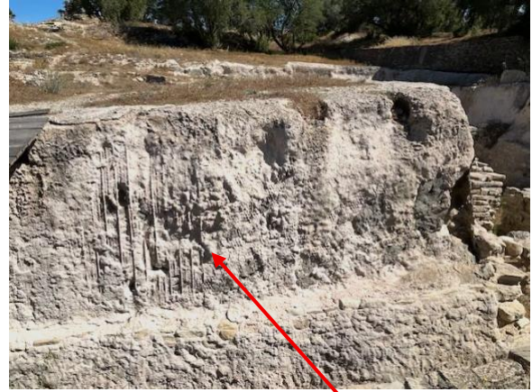
North face of Altar scarp showing exposed rusting metal mesh.
