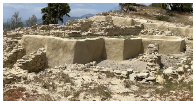
Example in Central Hillside of a new terrace with polypropylene netting enmeshed in mortar, spring 2024
