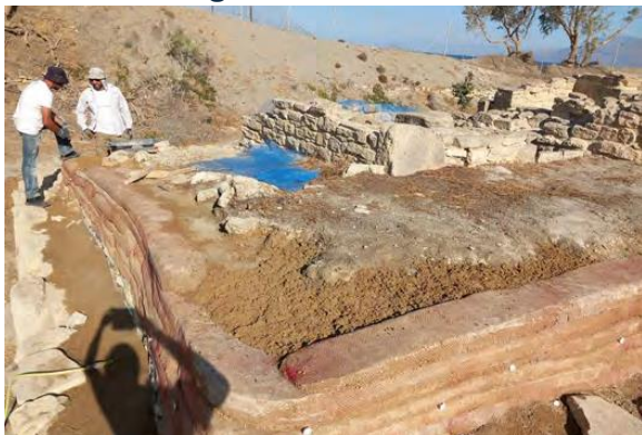
Packing mortar between soil scarp and adobe layers; Building W in background
